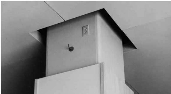
**Furring-Exterior Wall** Allow 6 mm (1/4") min. clearance between acoustical trim and intersecting exterior wall or column. Apply Acoustical Sealant as required.
