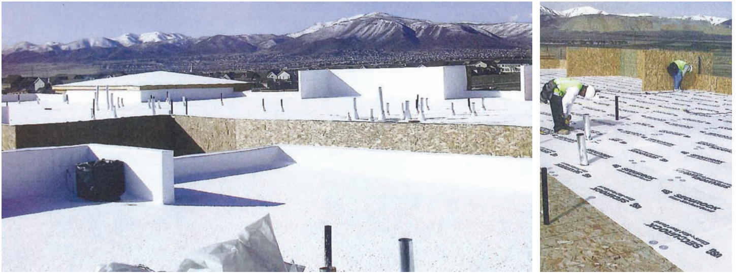
Apartment complex under construction in South Jordan, Utah
