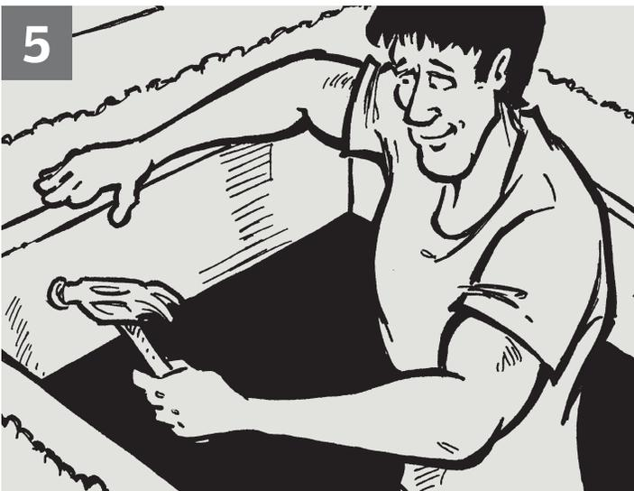
Frame the opening with headers and short rafters. As with the ceiling, use double headers and rafters if extra support is needed. Clean any sawdust or other debris from around the opening.
