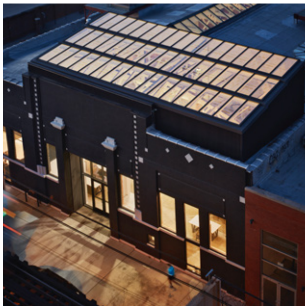
VELUX Modular System (VMS) Ridgelight and Step Longlight configurations, CoLaboratory, Chicago, IL
