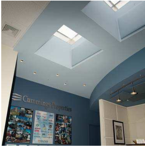
(2) CAP dome skylights with clear over clear acrylic
