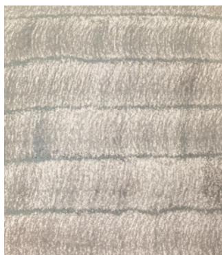
Proper Coverage on Insulation
