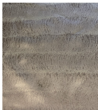
Proper Coverage on Membrane
