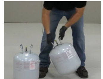
Shaking of A-side and B-side tanks
