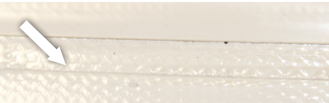
INCORRECT. HEEL DRAG CAN CAUSE DAMAGE TO MEMBRANE.
