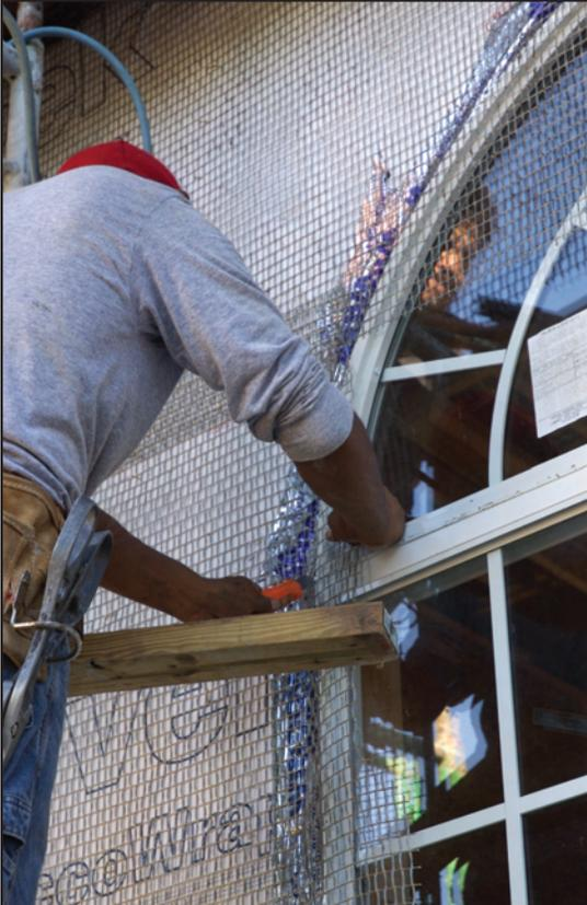
A light yet durable reinforcing lath that is corrosion-free and safer to handle. PermaLath is a woven fiberglass stucco lath that is a superior alternative to metal lath and stucco netting. Its performance has been proven in corrosive salt water environments, making for a rust-free stucco finish.
