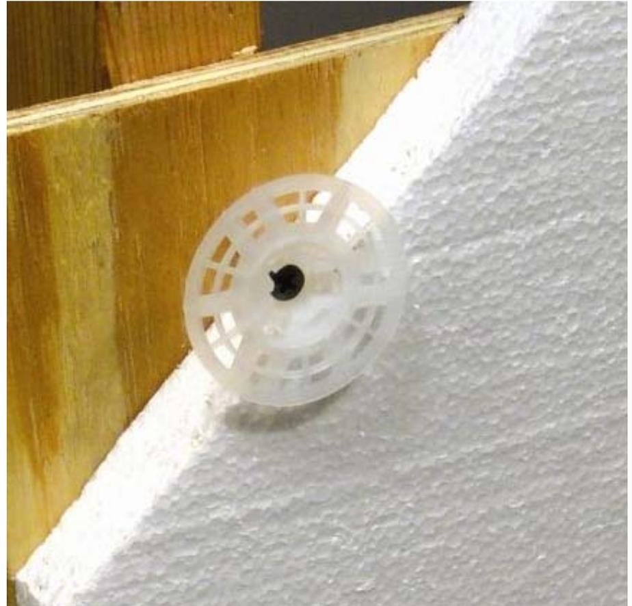
**NOTE:** Use caution when penetrating sheathing and avoid choosing a fastener that is too long and would cause damage to the services that can be present in the stud cavity wall.
