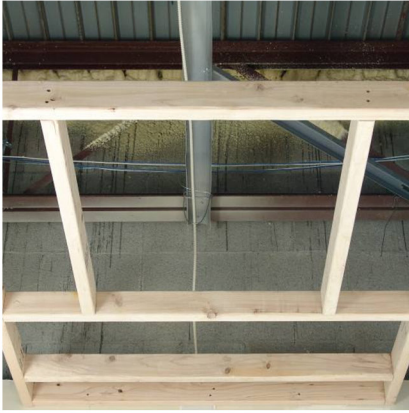
1. Frame out location of the panel.
