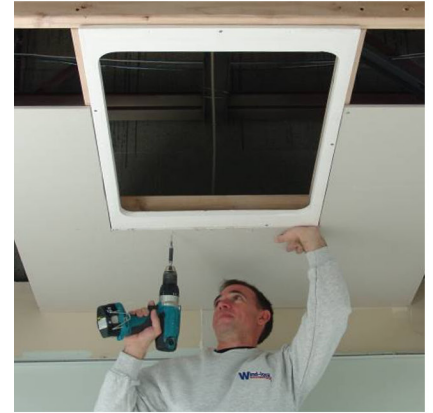
3. Hang drywall around the panel frame.
