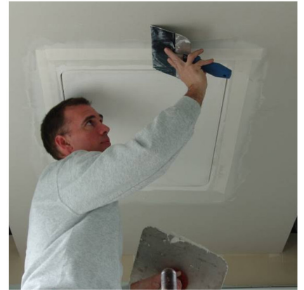
3. Smooth drywall tape and compound with a tapping knife.
