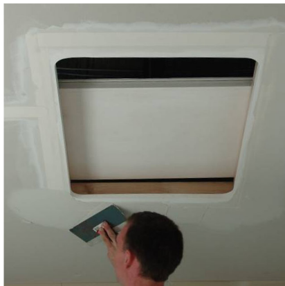
4. Apply second layer of mud and smooth with a tapping knife.
