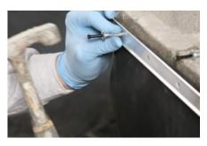
**Step 5**- Install the appropriate fasteners 6.0" – 8.0" (15.24 cm – 20.32 cm) apart penetrating the membrane and forming a compression seal to the substrate.
