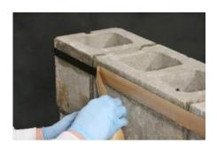
**Step 2** – The flashing must be applied at least 8.0" (20.32 cm) above the wall-to-footing transition.
