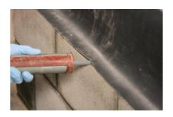
**Step 5**- Place a continuous bead of sealant within 0.5" (1.27 cm) of the outside edge of the brick shelf.
