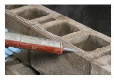
Step 2 - Apply a continuous 0.25" (0.64 cm) bead of Sealant within 0.5" (1.27 cm) of the edge of the mortar joint.
