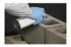
**Step 1**- Spray the substrate wall and the membrane with a Spray Adhesive/Primer and allow it to dry. Drying time is typically 2 - 3 minutes depending on ambient temperatures.
