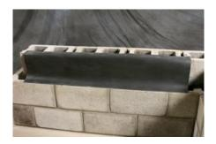
**Step 4**- Continue the membrane down the wall, continue over the wall-to-footing transition and continue out to within 0.5" (1.27 cm) from the edge of the brick shelf.
