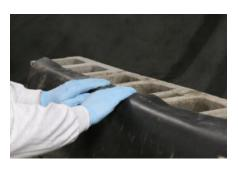
Step 3- Place the EPDM membrane at least 2.0" (5.08 cm) into the mortar joint and press into the Water Block Seal. Roll with a 1.5" (3.81 cm) roller to ensure complete contact.
