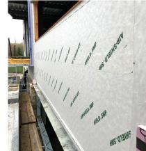
**AIR-SHIELD SMP** is a self-adhesive, vapor permeable, air/liquid moisture barrier that is designed to be fully bonded to the substrate without the use of an adhesive or primer.
