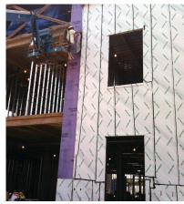
AIR-SHIELD is a strong and durable self-adhesive membrane that is protected by a special release paper. It remains flexible when surface mounted and will adhere to most primed surfaces.
