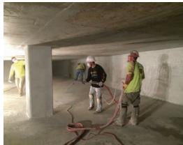
is a cost-effective solution to traditional resin-based linings and does not require a dry concrete substrate during application.
