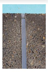
DECK-O-SEAL two-part, polysulfide-based joint sealant is a premium-grade, pourable, self-leveling sealant. It is a non-staining sealant that cures at an ambient temperature to a firm, flexible, tear-resistant rubber. DECK-O-SEAL is highly resilient and has excellent recovery characteristics after extended periods of compression or elongation.
