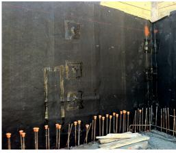
HYDRASTOP SA is an effective solution for applications where access to the site requires a pre-applied waterproofing membrane prior to pouring the foundation walls.
