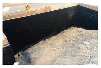
BACKFILLING Allow 24 hours for complete cure of membrane prior to backfilling.
