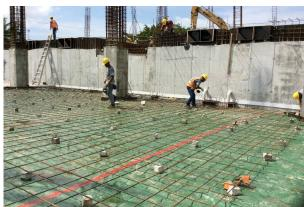
Low permeability, high strength and durability are all equally important selection and specification criteria for underslab vapor retarders/barriers. In fact, these characteristics are interdependent upon each other when it comes to preventing the migration of moisture into interior spaces. With **PERMINATOR**, you get the best of both world - superior puncture resistance coupled with one of the lowest perm ratings in the industry.
