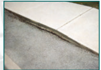
Ignoring expansion joints in pavement construction can lead to various problems such as cracking, chipping, and overall failure.
