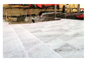
When a horizontal application meets a vertical application, ensure this overlap is a minimum of 1' (.3 m) from the base of the wall. Follow the end lap detailing instructions to address the overlap in this area.
