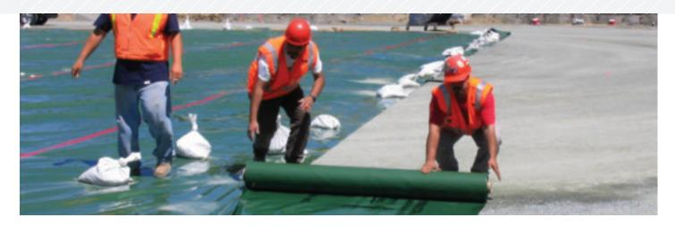
Uncontrolled water vapor through concrete slabs has cost building owners, designers and contractors billions of dollars. This moisture infiltration into structures contributes to the proliferation of mold, mildew and fungus that can lead to flooring system failures, including adhesive failures, warping, blistering and staining. In addition, water vapor migration carrying alkali can cause structural failure of the concrete when reinforcing steel is present.
