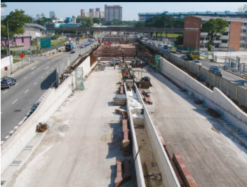
Immersed Tube Slide
