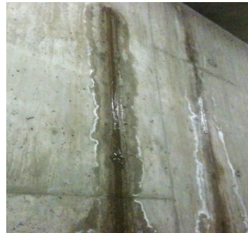
Leaking Joints
