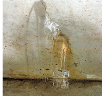
Leaking Joints
